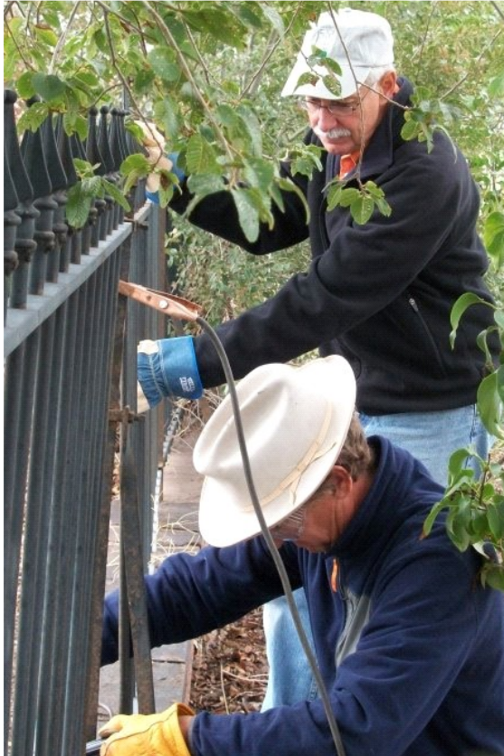
—Board members have a special work day to repair the wrought iron fence along Cerrillos Road.
