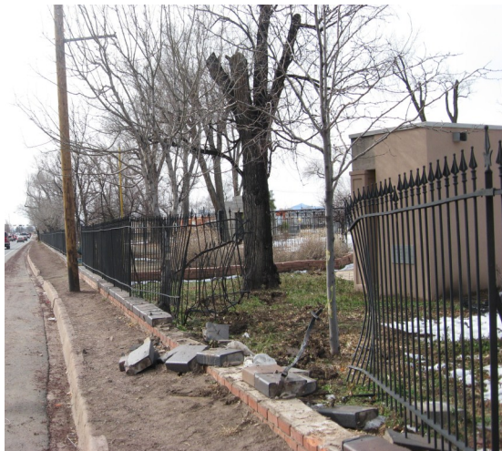
A driver who lost control of a car turning left from Cordova Road onto Cerrillos Road heavily damaged Fairview's historic wrought iron fence and at least two trees on Nov 30. Adjusters have not finalized a damage estimate, but it will be in the thousands of dollars..
