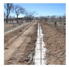
The wall is 950 feet long, goes five feet underground with solid concrete, three feet above ground with concrete, then topped with a 3-foot chain-link fence. Construction was closely monitored to ensure no damage was done to graves at the adjacent Odd Fellows Cemetery. A land swap also was negotiated with the cemetery's northern neighbor, the School for the Deaf, to prevent damage to graves closest to the fence line.
